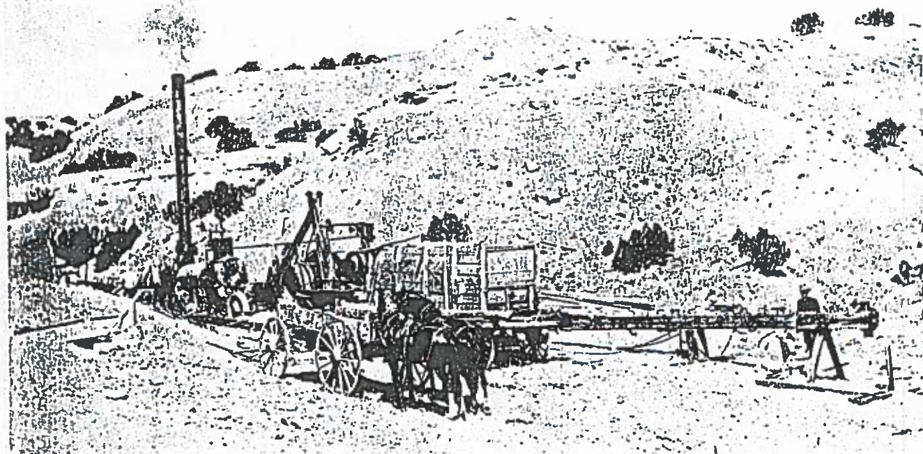
FIGURE 12.—Rigging up west of Asphalt Ridge at Uintah Development Company No. 3 well, sec. 17, T. 5 S., R. 21 E., Uintah County, Utah. T.D. 1,749'. Wooden mart on ground; boiler with steam up. April 26, 1913. C. J. Neal, operator.
