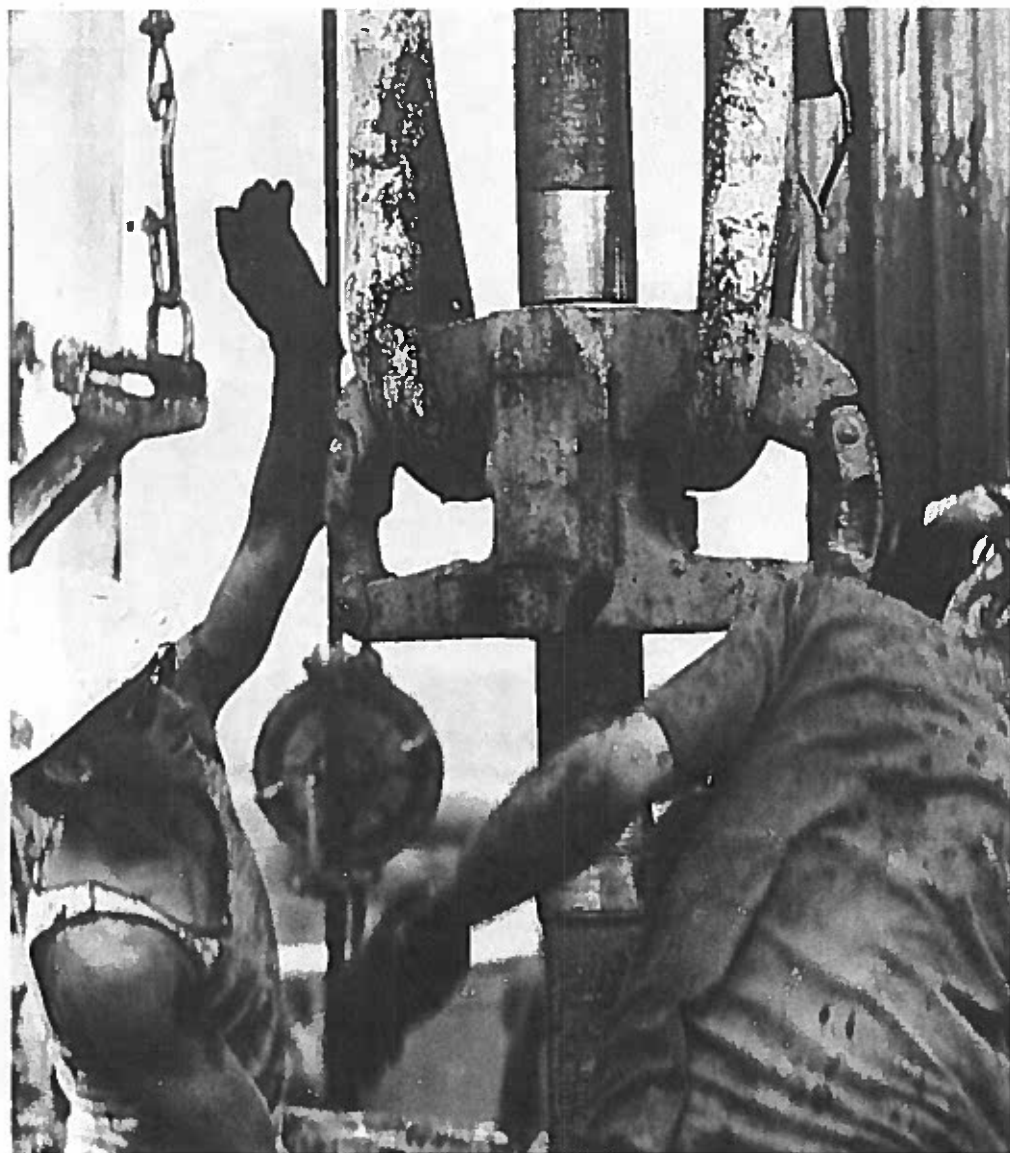
Drilling roughnecks use big power equipment to help handle pipe.
